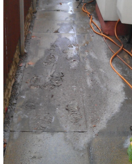
Figure 5: Foul debris residence side passage
