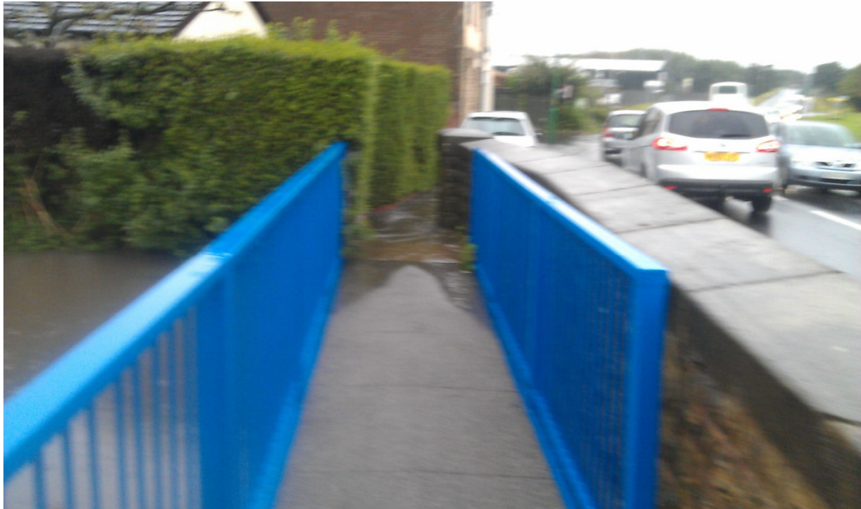
Figure 15: Dover’s Brook flooding into Sefton Lane, taken 24/09/2012
